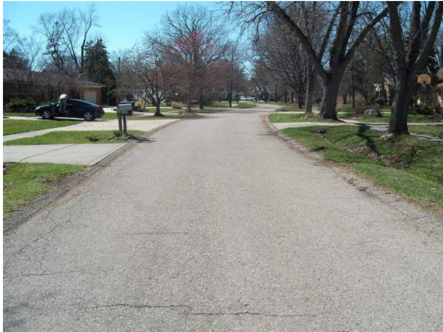
Redwood, El Dorado to Southfield Asphalt Condition Fair
