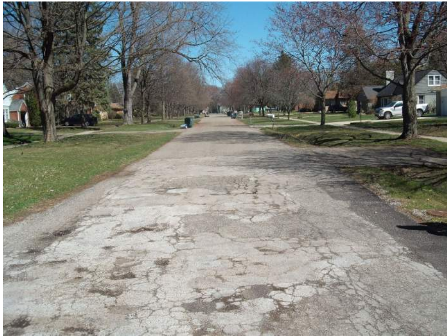
Saratoga, Bloomfield to Sunset Asphalt Condition Poor
