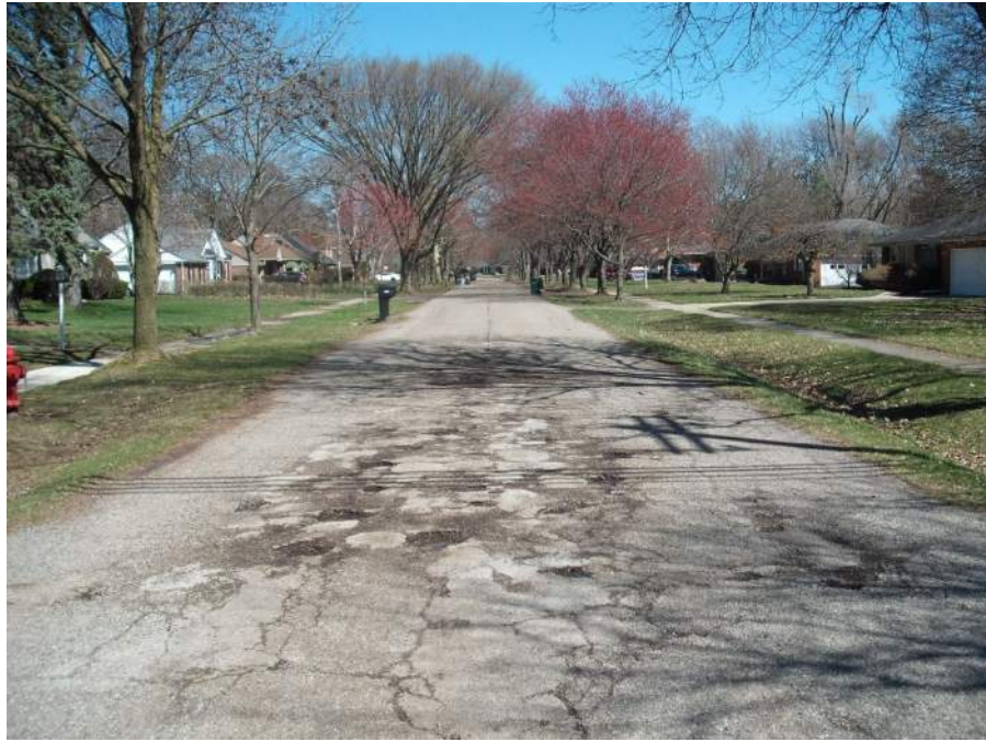
Cambridge, Santa Barbara to Bloomfield Asphalt Condition Poor
