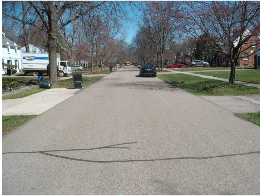
San Diego, Santa Barbara to Bloomfield Asphalt Condition Good
