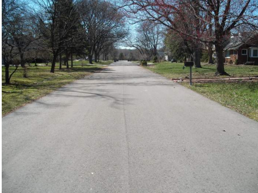
Wiltshire, Santa Barbara to Woodworth Asphalt Condition Excellent
